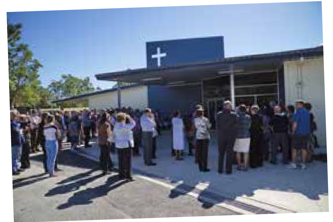
After years of prayer, visioning, planning, fundraising and working bees led by Senior Pastor Geoff Charles, Ministry Coordinator Cal Muggleton, and the leaders of Springwood Church of Christ, a new 600-seat church and community facility was officially opened on Sunday 21 April 2013.
